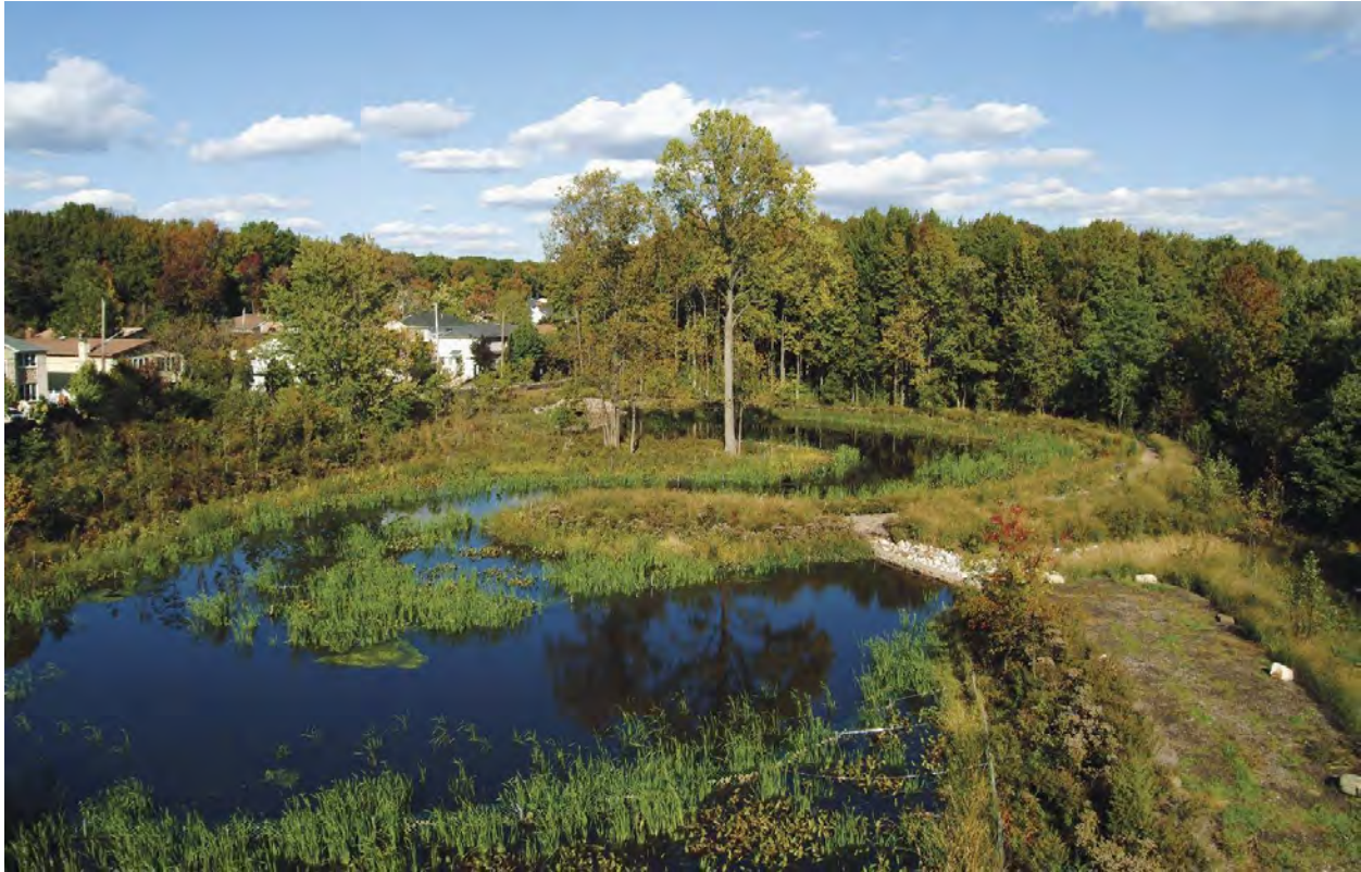
Figure 6-1: Constructed stormwater wetland in Staten Island, New York. Wetland design involves using biological process and high hydraulic retention times to treat stormwater runoff.
